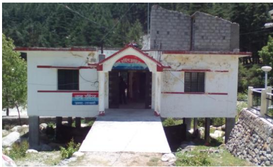
Figure 4. Single-story Police Station building at Harsil in Uttarkashi district built on stilts
