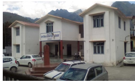
Figure 5. Double-story RCC Block Development Office building at Joshimath (Chamoli district)
