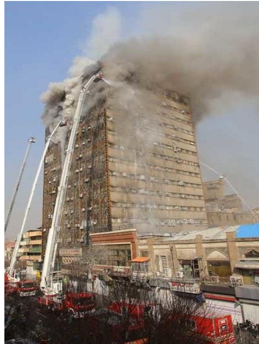
Figure 2. Recent fire incidents in high-rise buildings in 2017: The 17-story Plasco Building in Tehran which was engulfed by a fire and fully collapsed on January 19, 2017
