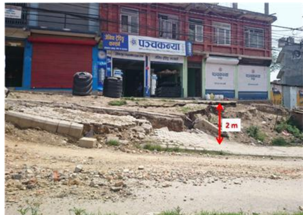
Figure 3. A typically observed ground surface fissure with NE-SW direction between Bhaktapur and Kathmandu.
