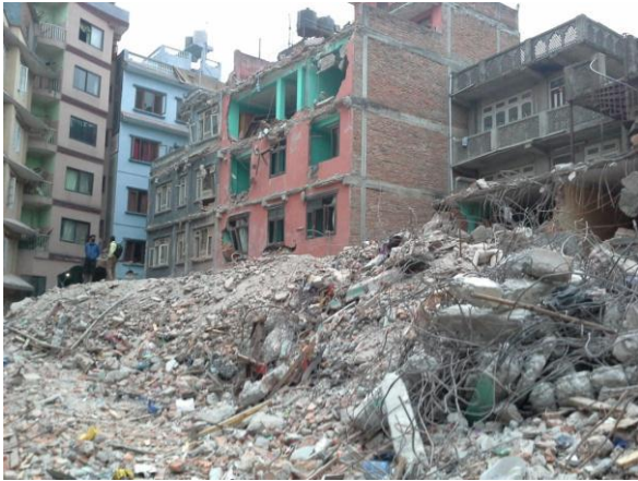
Figure 4. Severe damages to the building in Kathmandu.
