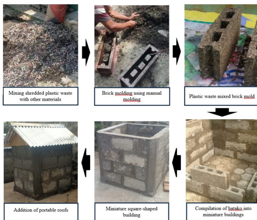
Fig. 1. The method of creating tiny structures out of plastic trash
