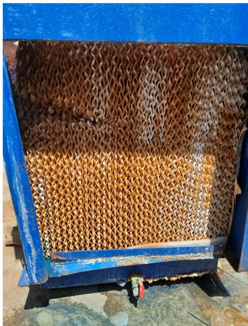
Fig. 3. Partial onset of fouling due to the formation of carbonate
